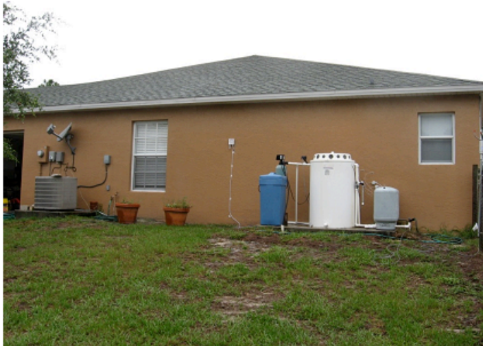
(a) South face of house
