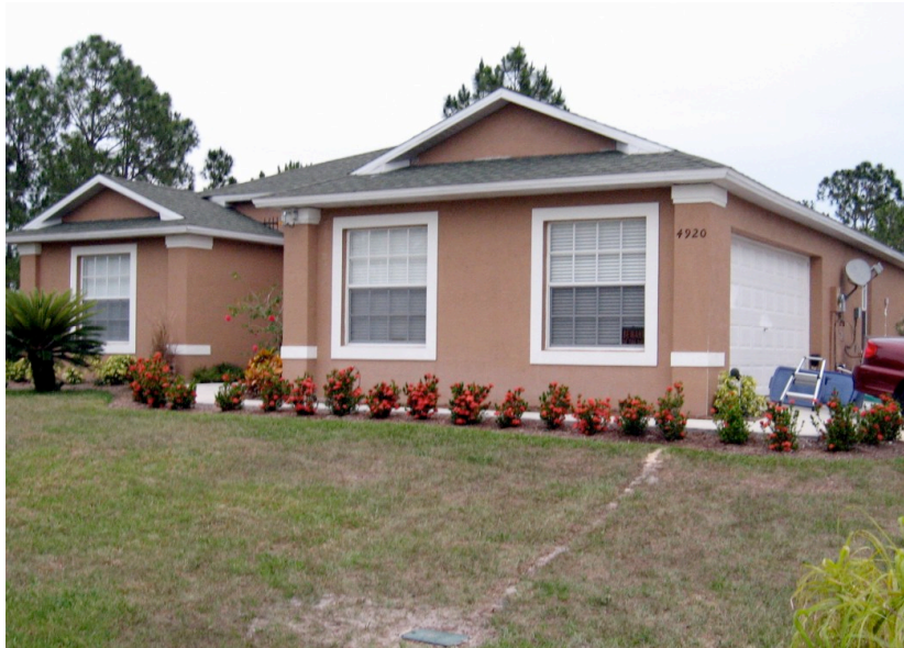
Figure NF-1 - Photograph of the one-story house with 3 instrumented cracks
